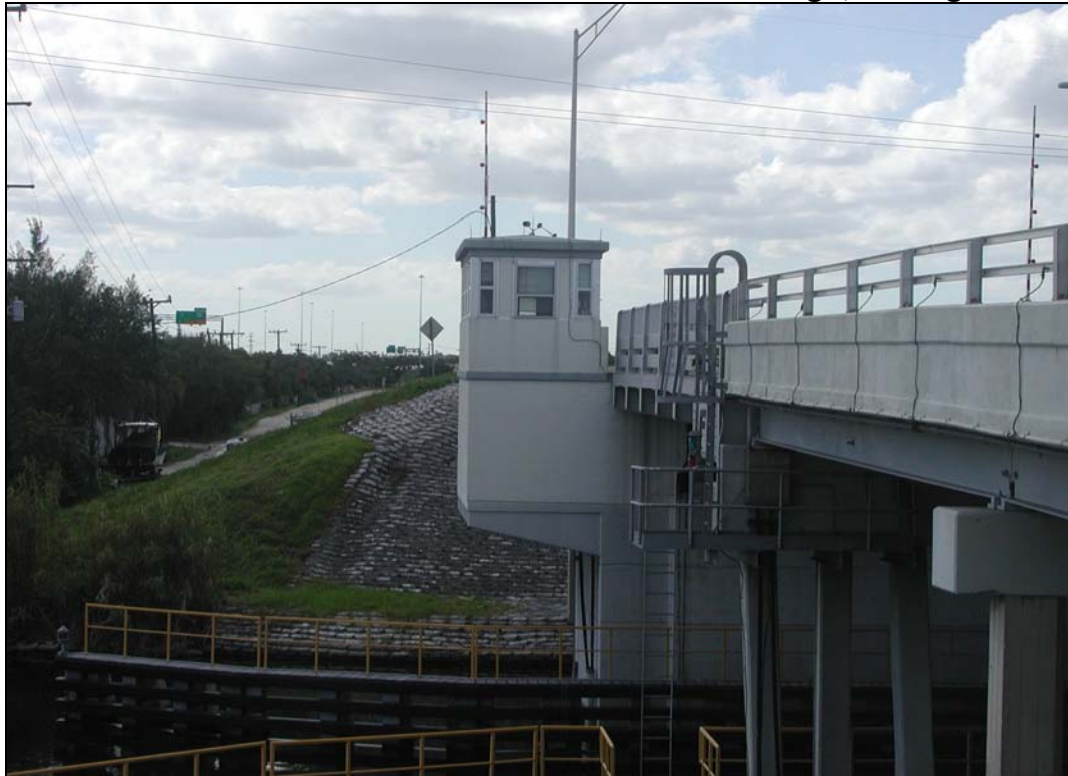
Figure 9-11 Tender Station of the South Fork of New River Bridge, Facing West
