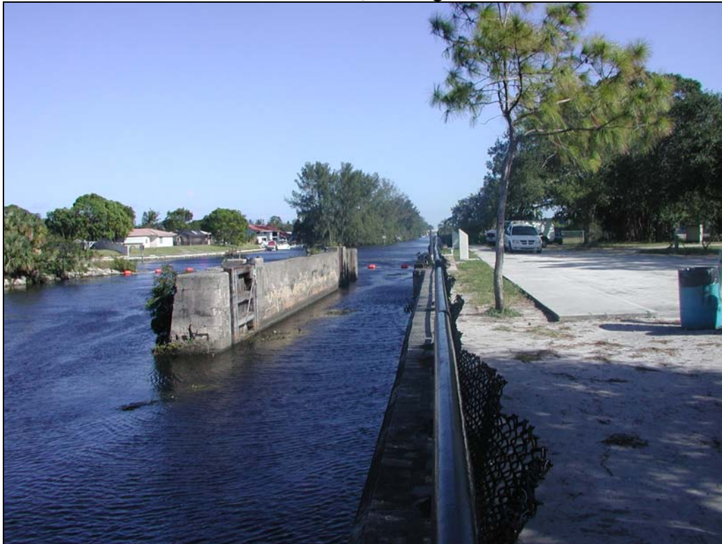
Figure 9-4 Sewell Lock, Facing East
