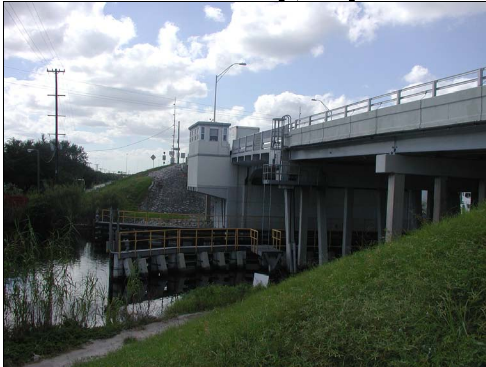
Figure 9-10 South Fork of New River Bridge, Facing Northwest
