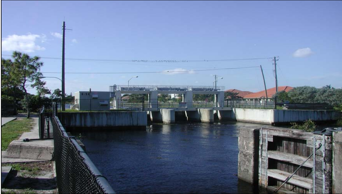
Figure 9-6 G-54 Sluice Dam, Facing West From Sewell Lock
